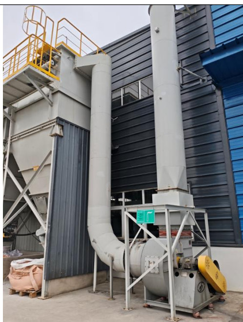
废气排放口标识牌-粉碎除尘DA004
